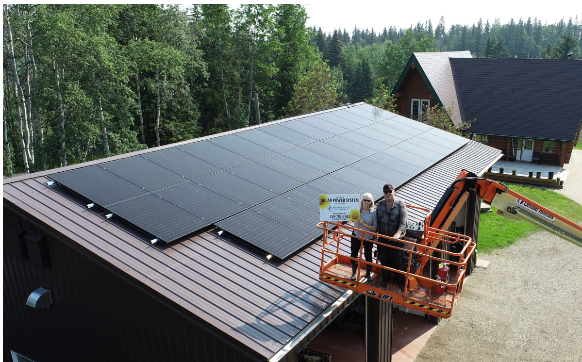
A phase 2 installation of 6.9 kW for a total array size of 15.4 kW. Near Fort St. John, BC.
