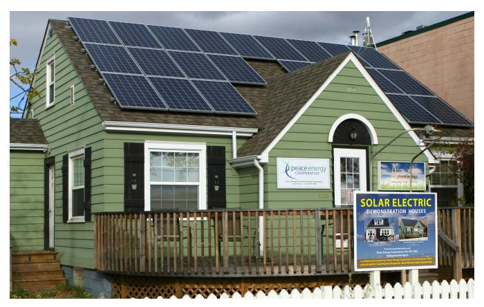
Peace Energy Cooperative has installed a grid-tie solar demonstration system at their Dawson Creek, BC offices. Commissioned in November 2013, the building achieved net-zero energy usage after its first full year of operation, and has continued to produce more electricity each year than it uses: no electricity bills for six years straight!
