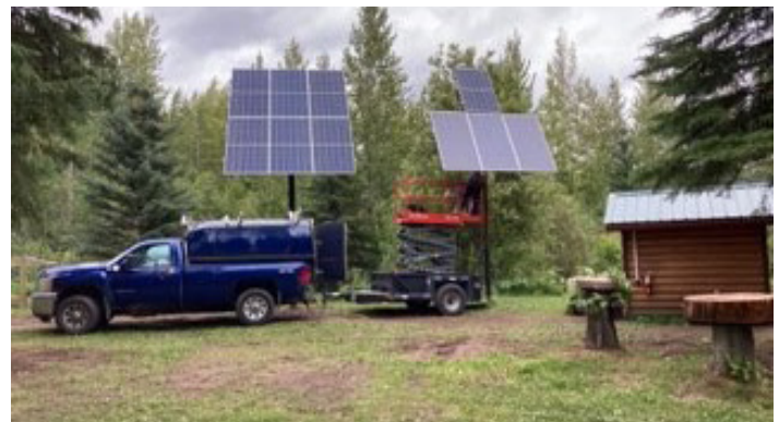
We have just designed and supplied an off-grid 2.9 kW solar upgrade for the off-grid system at the Pat O'Reilly Outdoor Environmental Study Centre at Gwillim Lake, BC.
