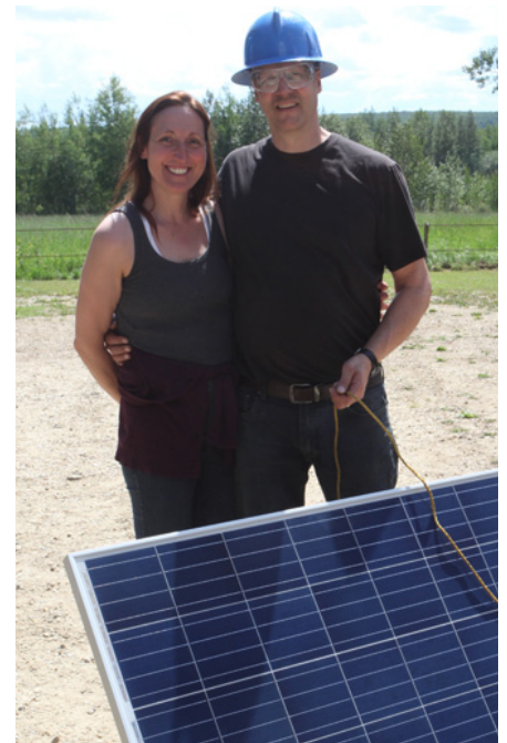
Greg and Joanne Dueck were there to help with the solar install at the Demmitt Hall in Alberta this summer.
