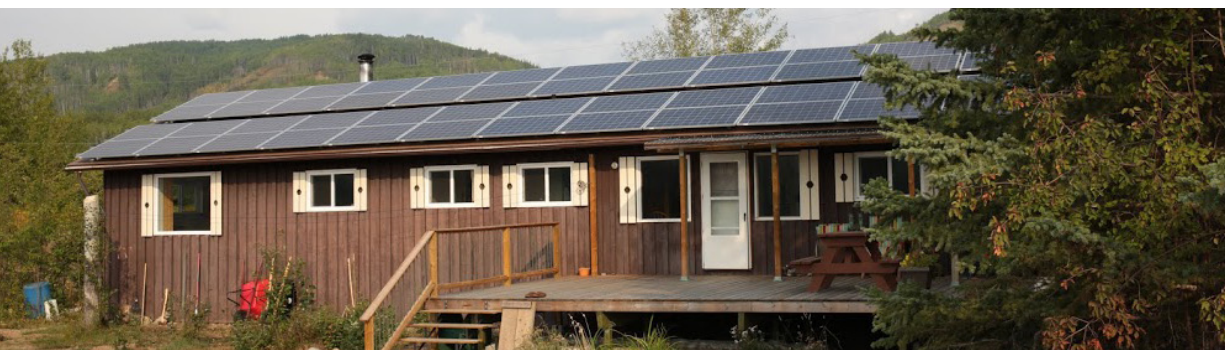
This 12 kW solar array on the Armitage home in Hudson's Hope, BC, will provide all the energy this family needs for next half century. (Array designed and installed by Peace Energy Cooperative.)
