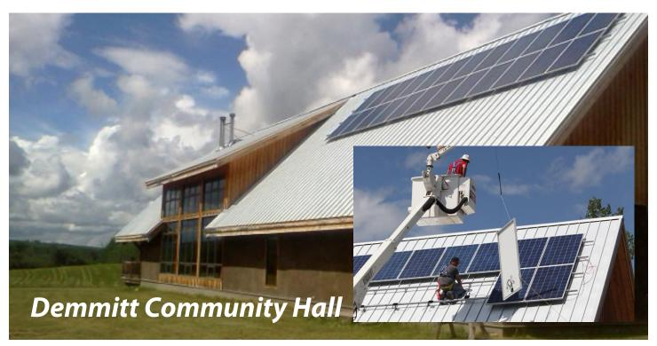
**Description:** South-facing roof provides excellent solar exposure with essentially no shading. The high, steep steel roof angle is good for shedding snow and increasing winter solar gain, but required installation by bucket truck (inset) which was slower and more
