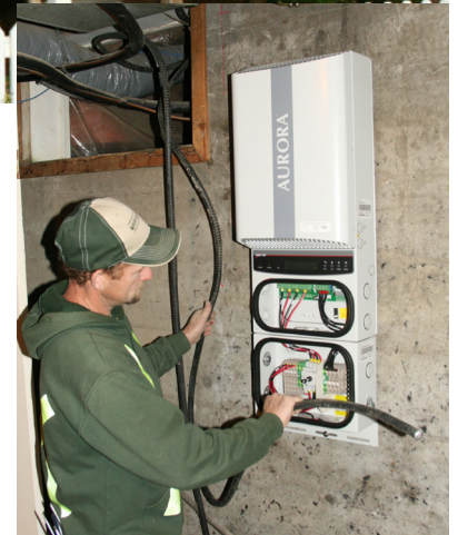
Ron Moch of Moch Electric Ltd. installing the 5 kw inverter that feeds solar power to the building and the grid.
